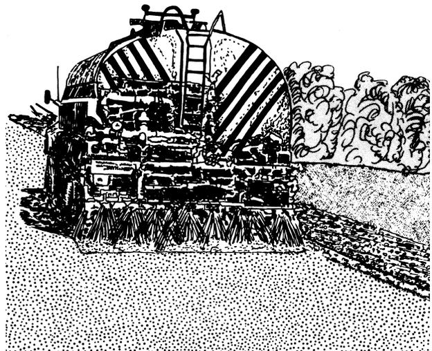
**When applying liquid calcium chloride, overlap the centerline which carries the most traffic. Avoid runoff or puddling. If areas are left uncovered by poor driving of the distributor, stop and add water before beginning to spread again.**
