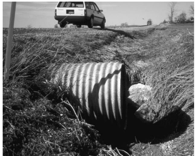
*Erosion, a sign of inadequate capacity, has undercut the end of this culvert pipe.*
