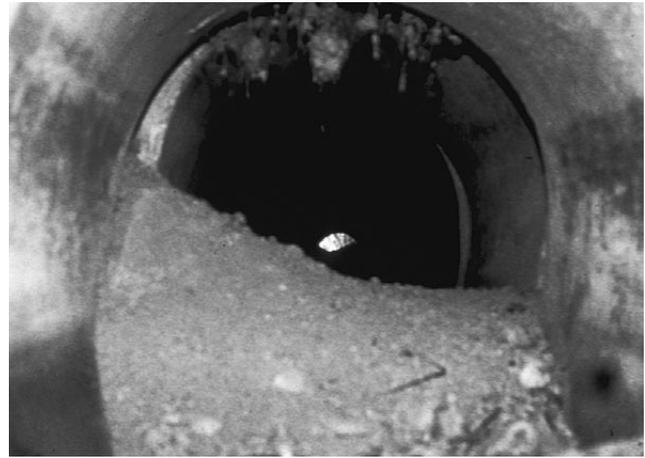
*Silt filling this culvert drastically cuts flow capacity.*
