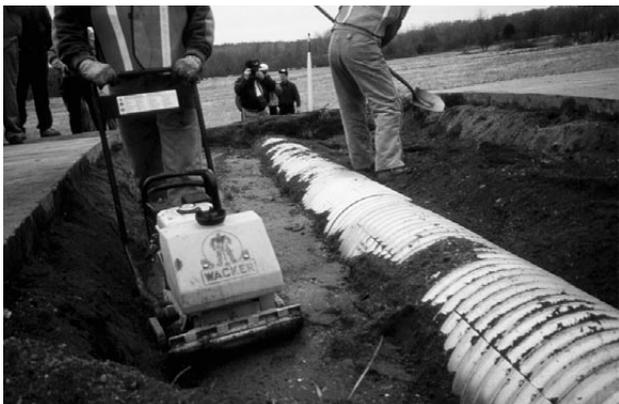
*Adequate compaction is essential to culvert installation. Hand tamping is often best.*
