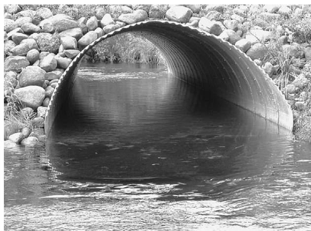
*This beveled or mitered culvert is set sufficiently low to minimize upstream channel impacts, will allow fish to pass because of good depth and low velocity, has adequate size to pass flood flows, and good erosion control (2:1 side slopes, riprap, vegetation).*
