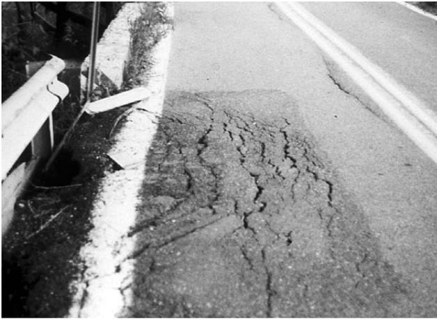
*Cracks and settling in asphalt indicate a failing culvert.*
