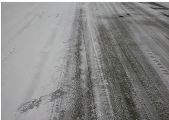
*Photos taken during an anti-icing pilot De Pere conducted two years ago show the contrast between the brine-treated half of a city street on the right and the untreated side. Application at the onset of a storm helped break the bond of snow and ice to pavement, making clean removal easier.*
